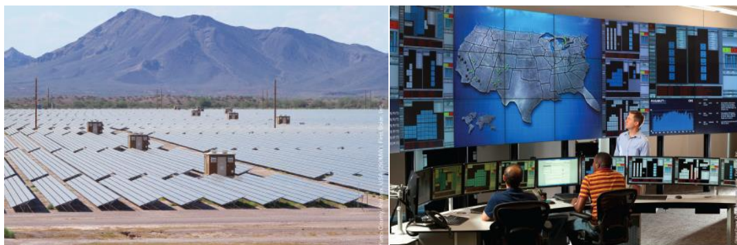
Figure 29 (left): First Solar's Yuma County-Arizona, 290 MWp CdTe PV power plant with grid-friendly plant control and (right) Operations Center in Tempe, Arizona, controlling over 2,000 MWp of solar power plants operating in the USA 69 .
