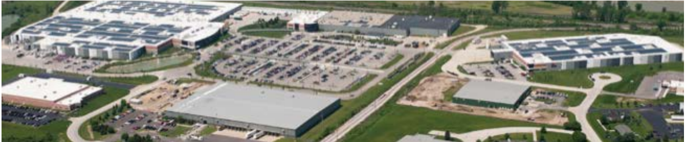
2.75MW AC Rooftop and Ground-Mount PV Installation at First Solar's Perrysburg, Ohio Manufacturing Facility.
