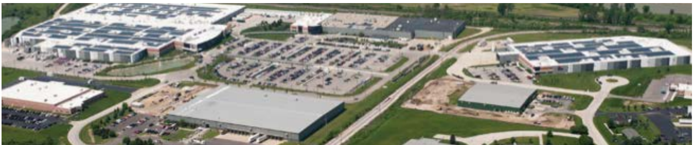
2.75MW AC Rooftop and Ground-Mount PV Installation at First Solar's Perrysburg, Ohio Manufacturing Facility.
